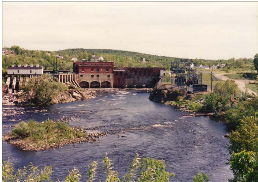
Photo of the Power Dam at Milltown, NB. Photo taken in 2008, looking upstream
